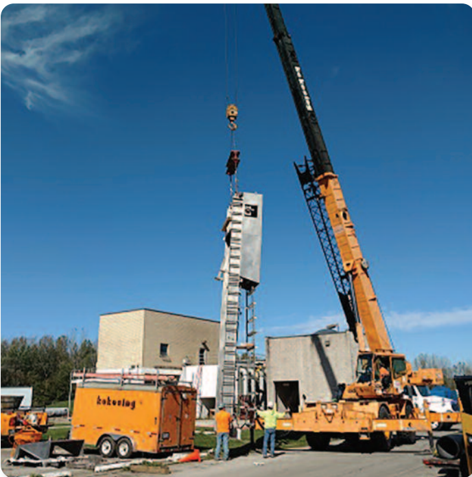
Lock Link Screen Installation New Castle Indiana
