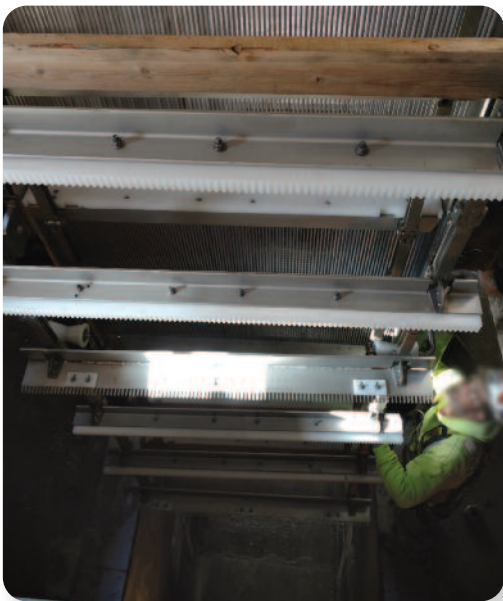
Lock Link screen arrives fully assembled or with bolted modular pieces for deep channels.
