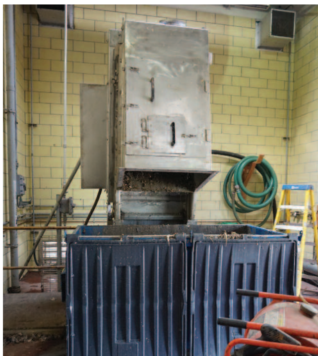
Thanks to the Lock Link screen, a 3 cubic yard dumpster replaced the bucket.
